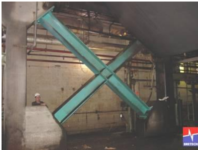
Figure 5: Structural modifications to minimize machine vibration Source: http://www.bretech.com , accessed on July 14, 2009.
